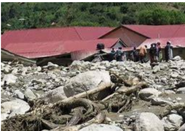
Mines and Tronder Hydro Plant in Kasese Destroyed by Floods May 2020
